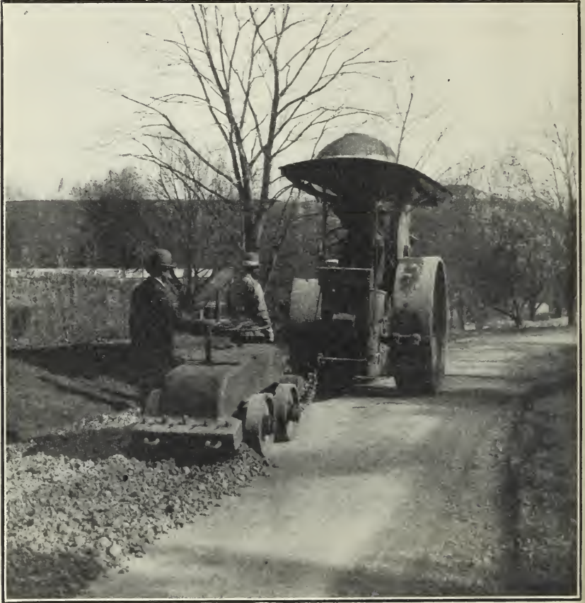
FIG. 3.—Another type of scarifier.
